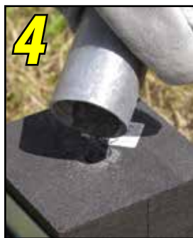
4 Place a small amount of starting powder in the ignition pocket.
