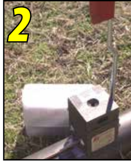
2 Position conductor and mold onto pipe.
