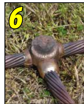
6 Remove weld and clean mold before making next connection.
