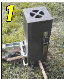
1 Position cleaned conductors in mold.
