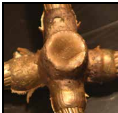
Image 3: A worn or incorrect mold was used, allowing leakage around conductor. The fill in this connection is sufficient to make it as acceptable.
