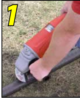
1 Clean pipe before making weld.
